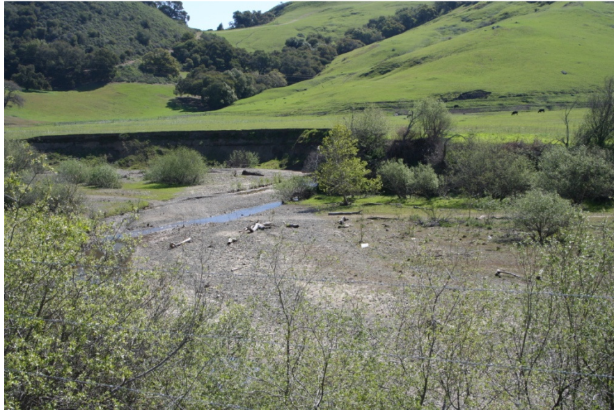
Stream bank erosion in oxbow area of Santa Rosa Creek in the upper watershed.
