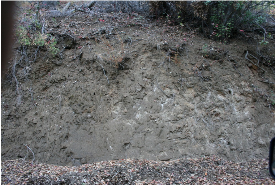
Upslope road erosion in upper watershed along Santa Rosa Creek Road.
