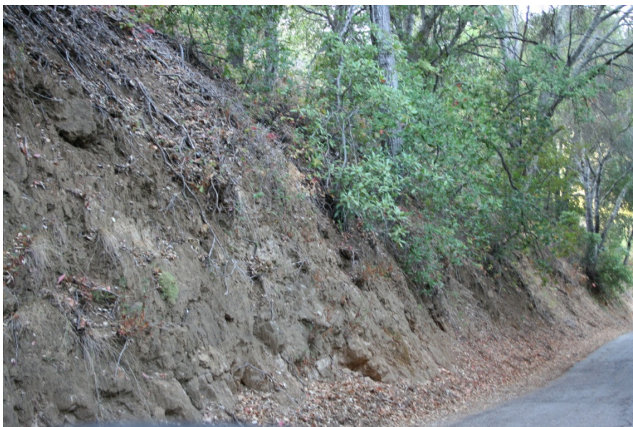
Upslope road erosion in upper watershed along Santa Rosa Creek Road. Site underneath tree canopy and would not have been mapped using GIS and aerial imagery.
