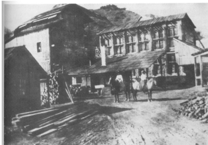
Huge buildings over the shafts of the Oceanic Mine. Taken about 1917. The outbuildings held blacksmithing forges, the office, crushers, etc.
