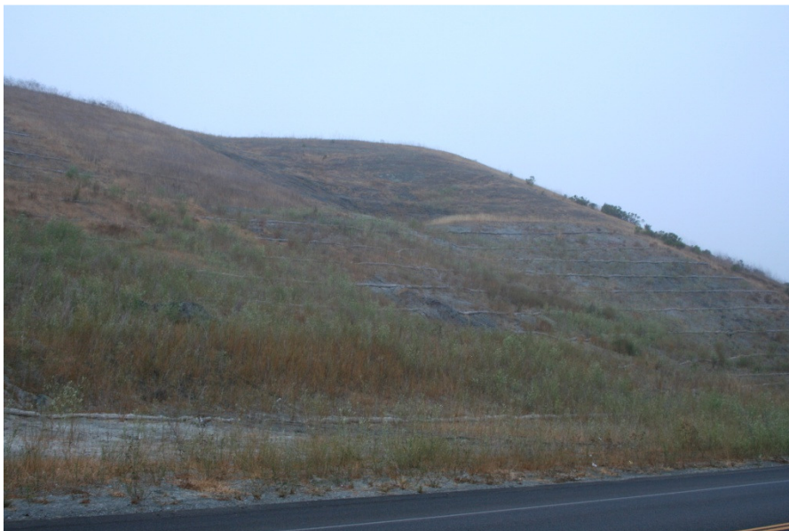
Road erosion along State Highway 46 in Perry Creek Watershed.
