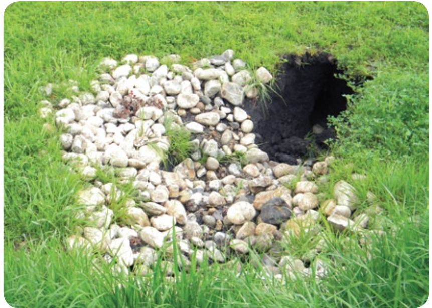
Rock rip-rap placed at the outlet of a culvert
