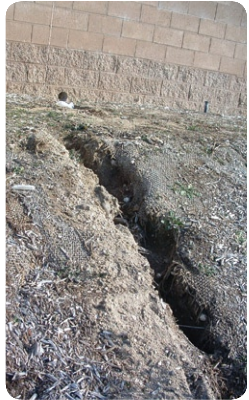
A rill forming at the outlet of a pipe
