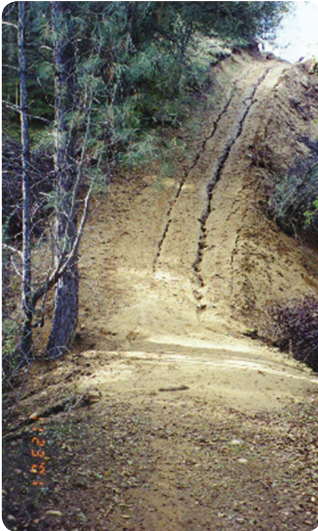
Rills forming along an unmaintained dirt road
