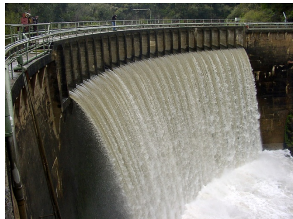
San Clemente Dam – Carmel River
