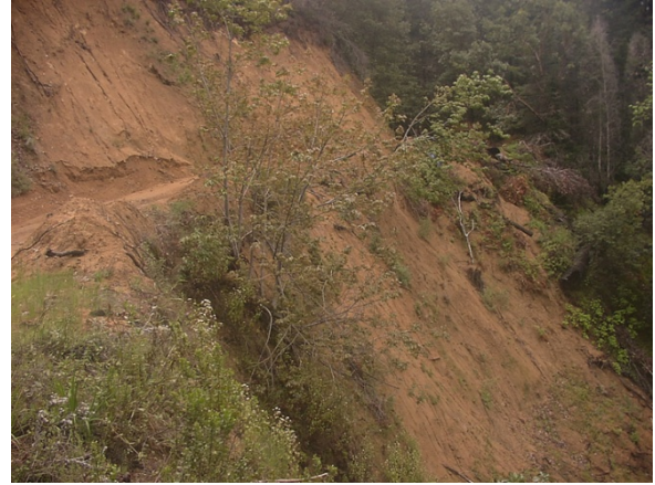
Little Sur River – Road Cut
