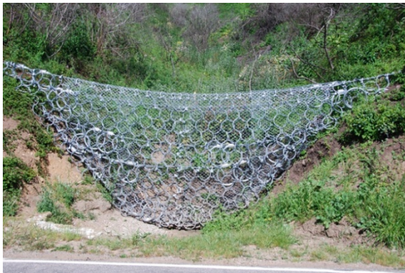
Big Sur Coast – Post-Fire Debris Control Structure
