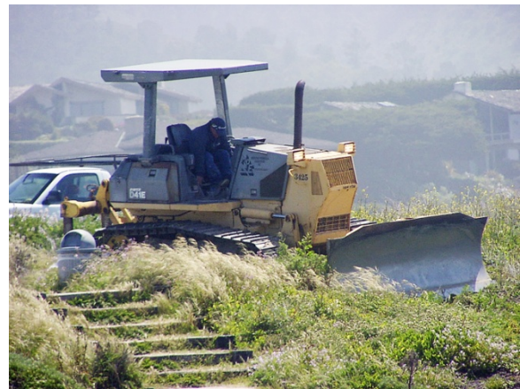
Flood Control Work – Carmel River Estuary
