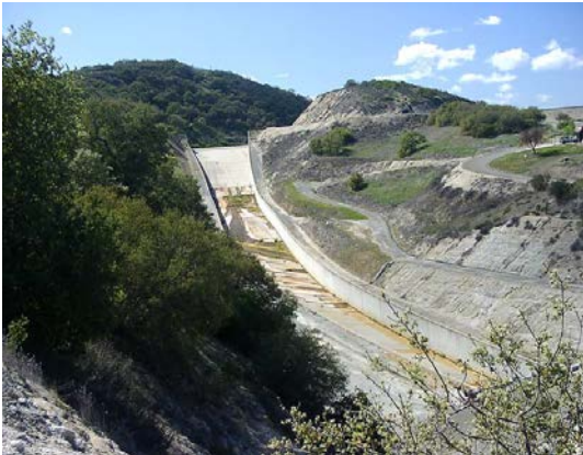
San Antonio Dam
