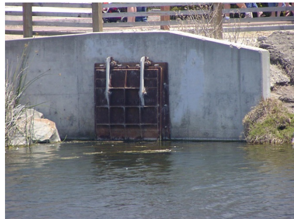
Pismo Creek Estuary - Storm Drain
