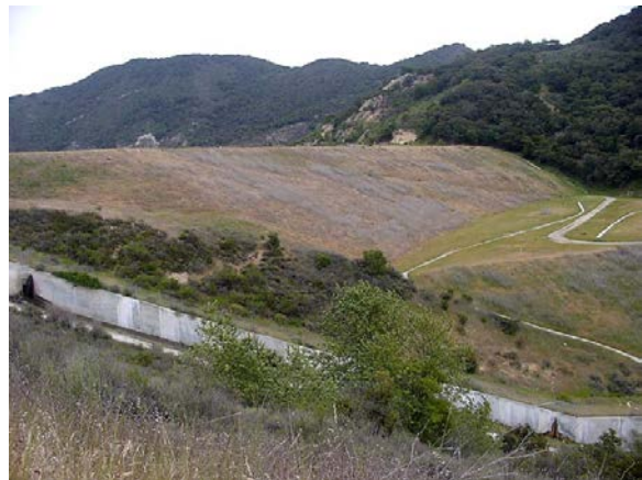
Arroyo Grande Creek - Lopez Dam
