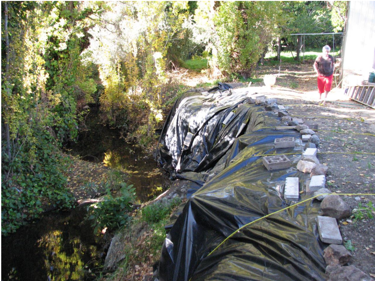
Figure 7. Example of Bank Stabilization in San Luis Obispo County.
