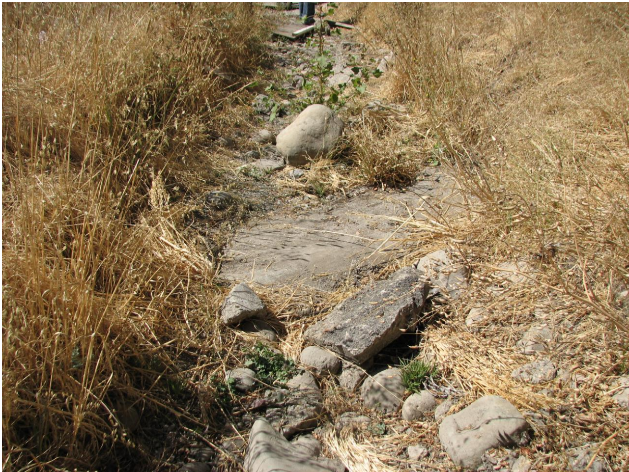
Figure 8. Example of Utility line protection in San Luis Obispo County.
