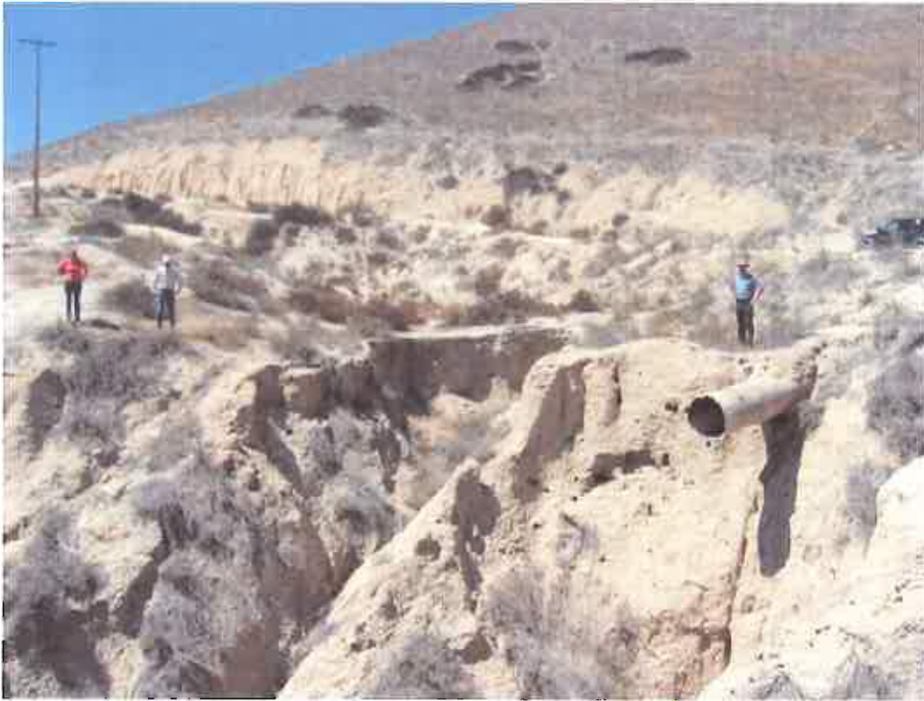
Another large eroded gully caused by poor road design and inadequate storm drainage system
