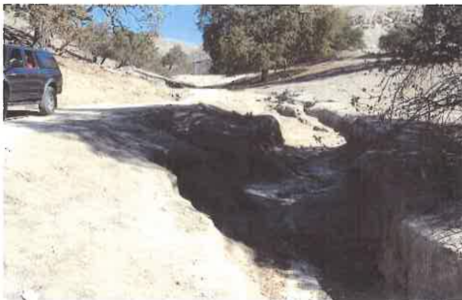
Drainage from ranch roads has caused soil erosion
