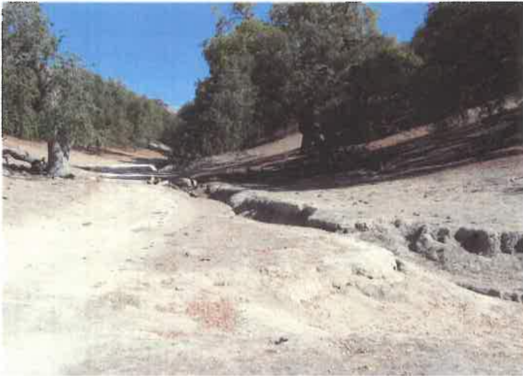
Ranch roads in draws, ravines, and valleys can become a conduit for storm flow, accelerating and concentrating flows that cause soil erosion and gullies
