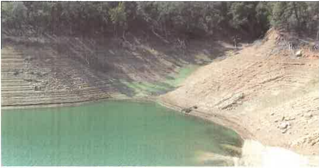
Step like soil erosion below “high water mark.” Erosion at right side is in excess of 6 feet in depth.
