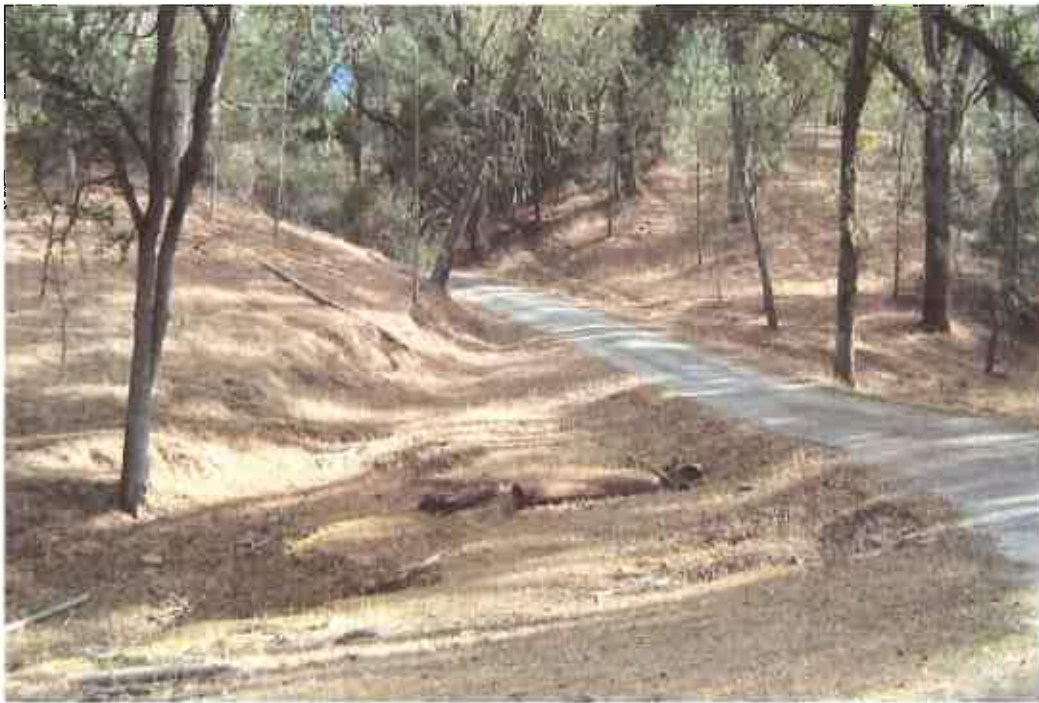
Ranch roads that are "out-sloped" are less likely to cause concentrated flows or soil erosion
