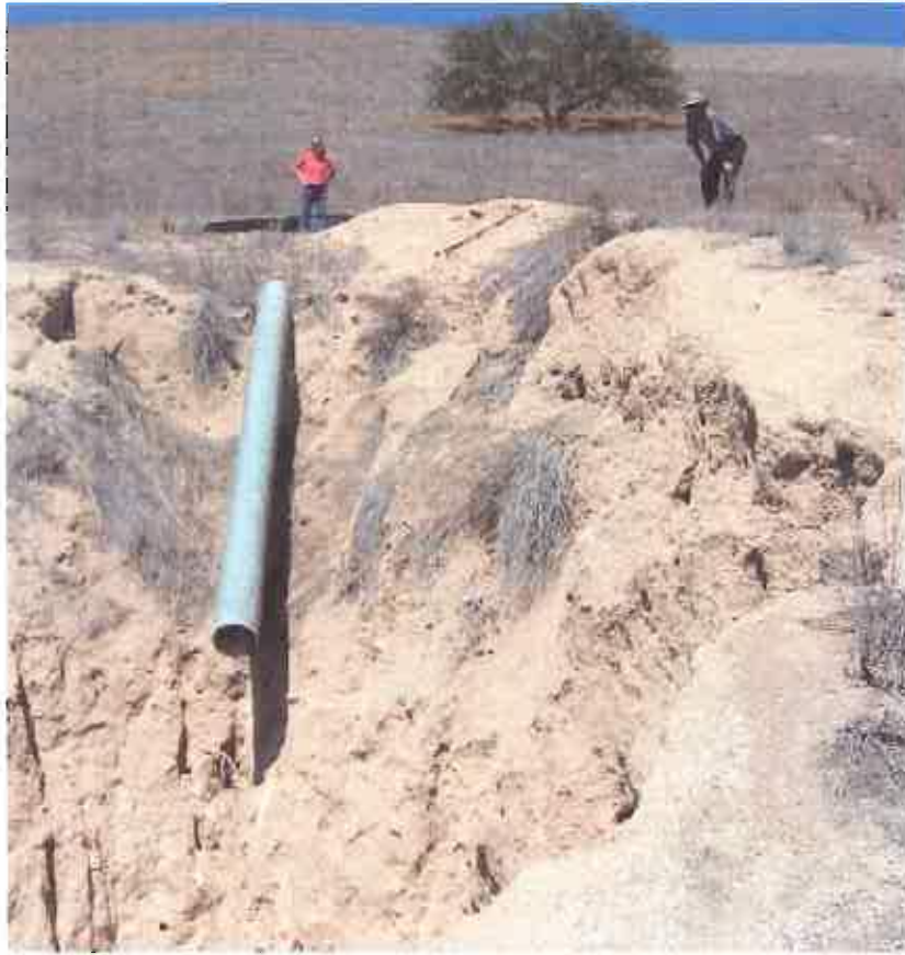
View of erosion and exposed culvert pipe
