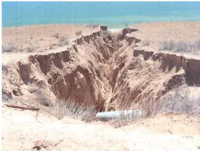
Undersized culverts, blockages by debris and poor road drainage are causes of erosion
