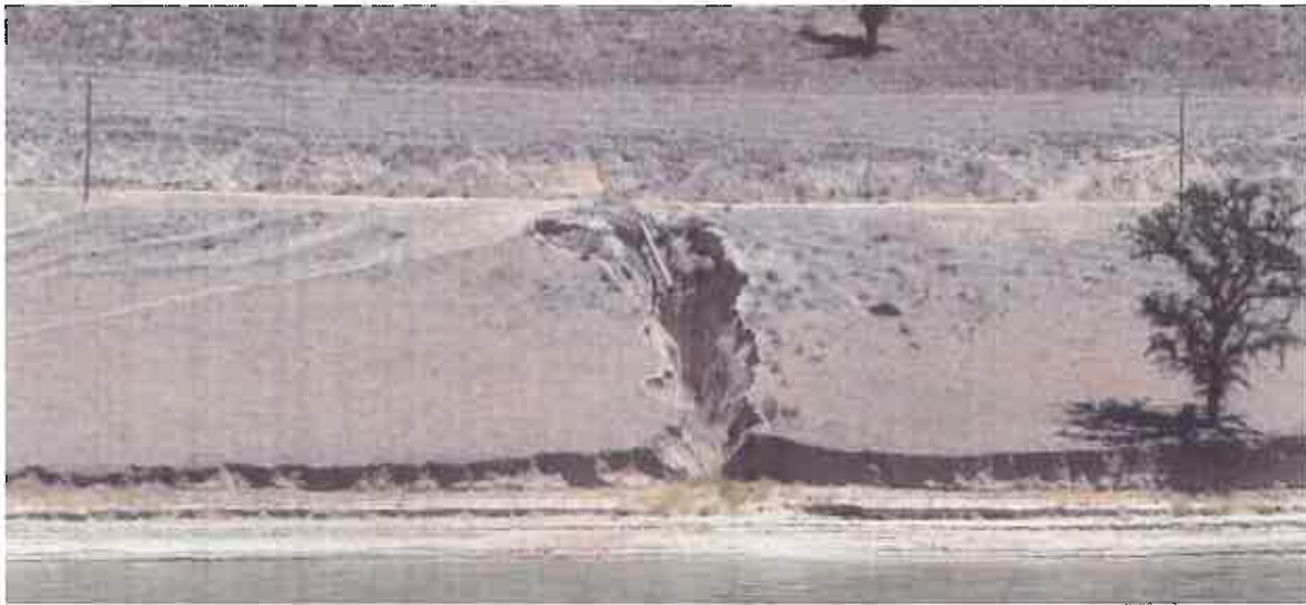
Road drainage is second greatest cause of erosion on the lease properties
