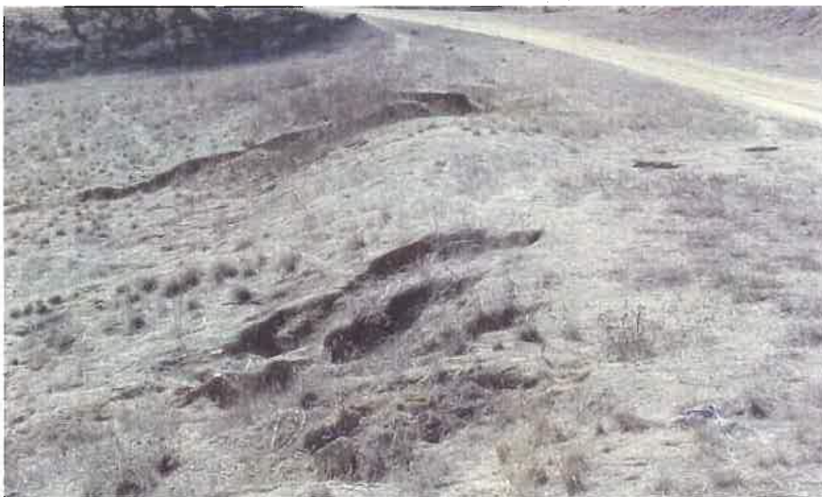
Example of erosion caused by squirrel holes
