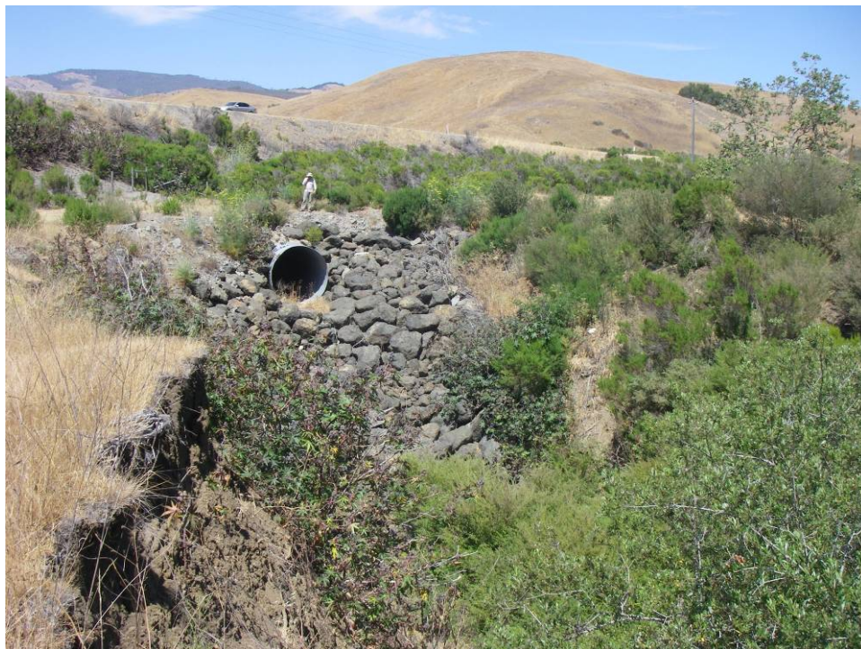
Figure 4-14. View looking upstream at a large, 7-ft diameter culvert that passes beneath Highway 46 and drains into Green Valley Creek.
