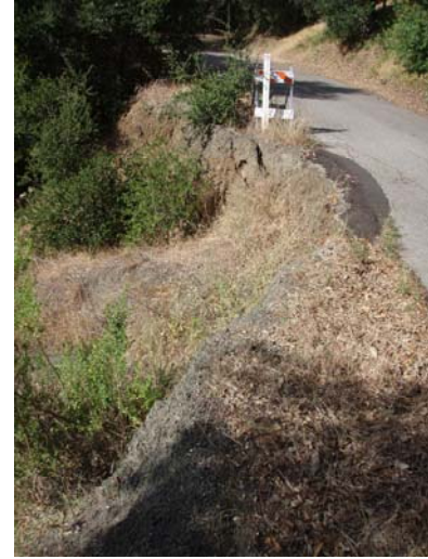
Erosion at Santa Rosa Creek Road
