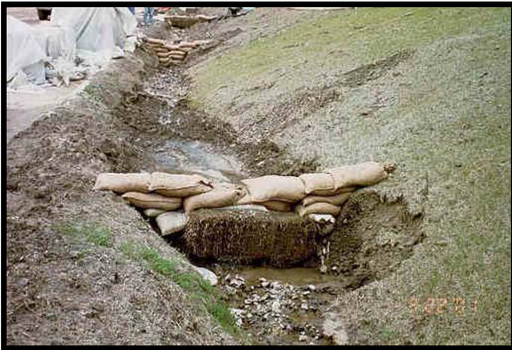
Example of Improper Use of Hay Bales and Sand Bags in Gully Hay bales, silt fences, and Sand Bags used in gullies often cause worse erosion.
