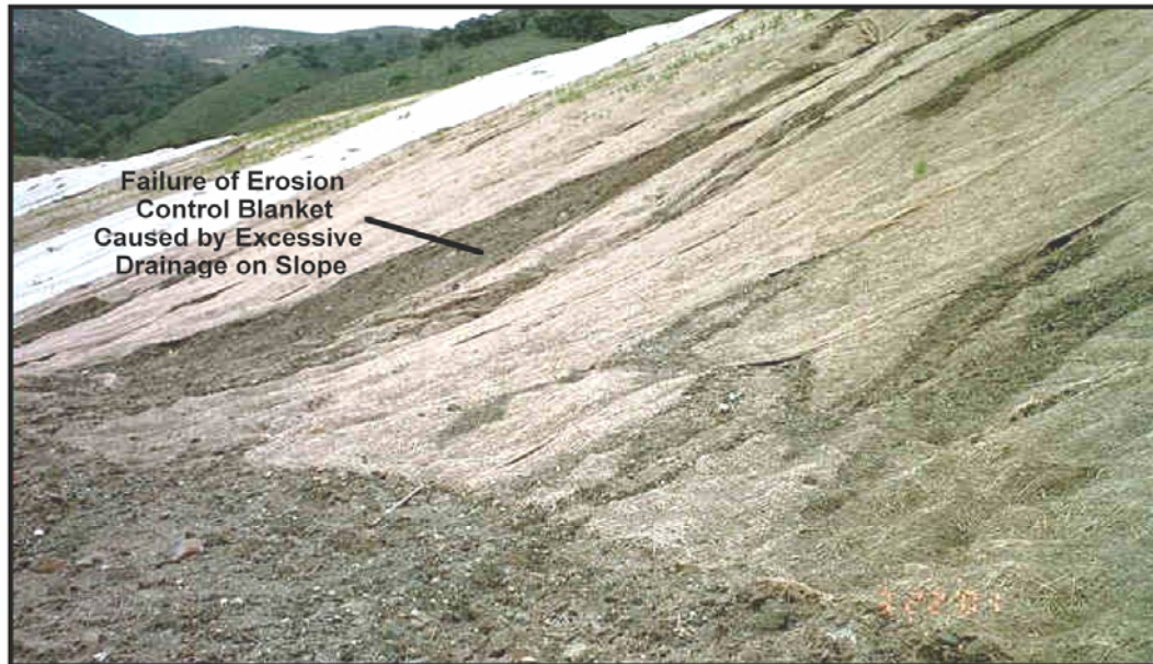
Partially Failed Erosion Control Blankets from Excessive Runoff Runoff should NOT be permitted to concentrate at top of blankets
