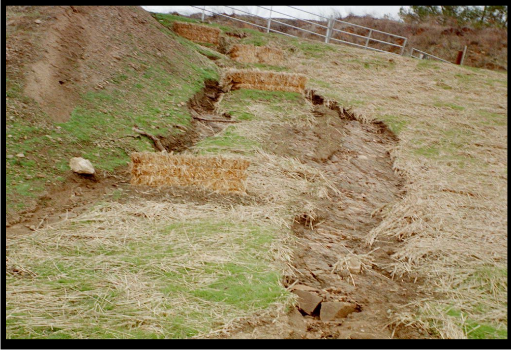
These two gullies were formed by misuse of hay bales. Placed in the path of runoff from an adjacent road, the hay bales interrupted sheet flow, accelerating erosion on either side.
