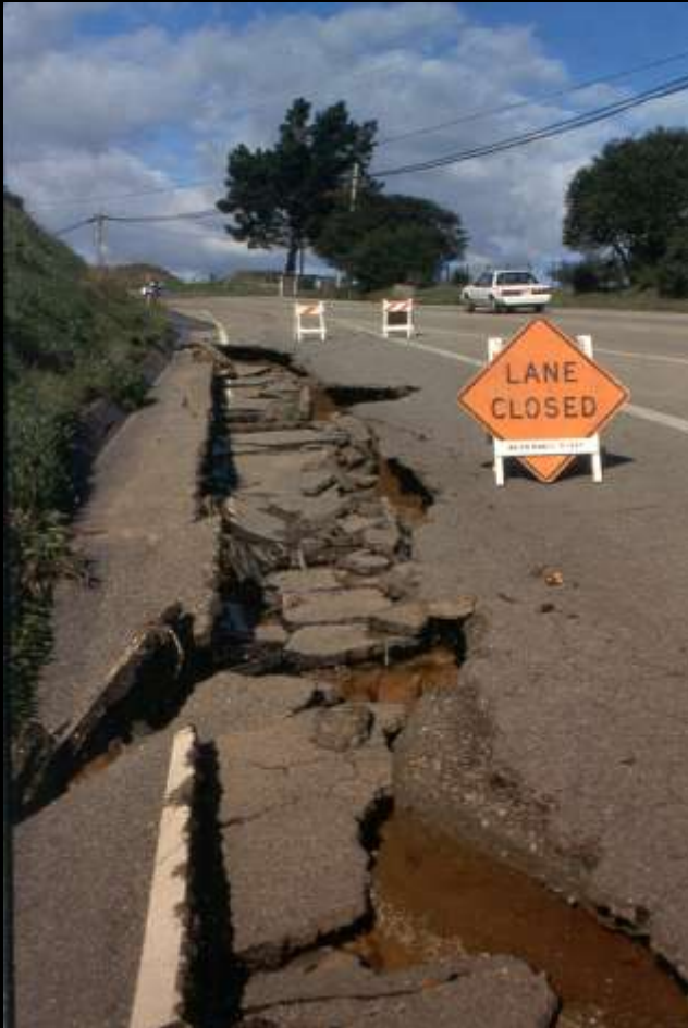
Elkhorn Road turn lane damage from farm runoff
